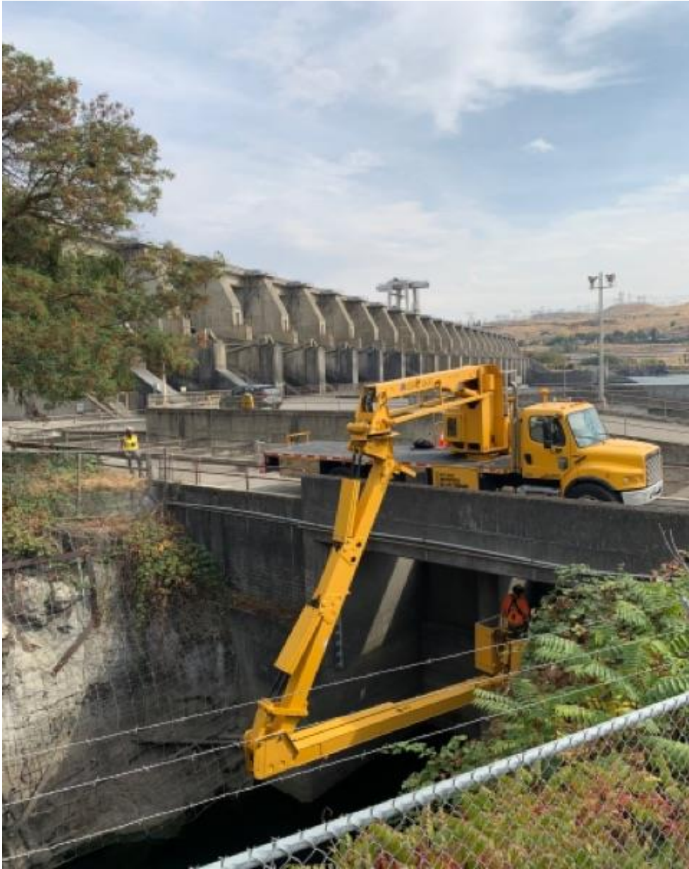
Bridge inspection at North Fishway.
